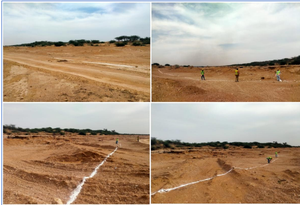
Figure 7: Photographs of marking the ROW using limestone at Mazarani Dam Site
