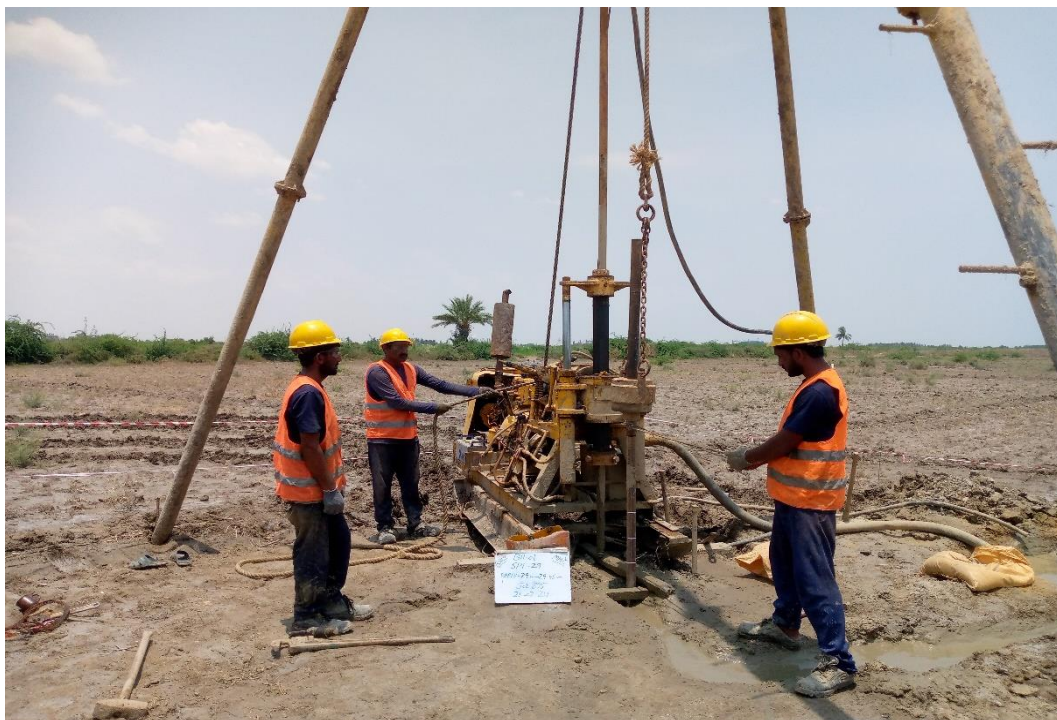
Photo-1: Performance of Standard Penetration Test at the location of BH-01.
