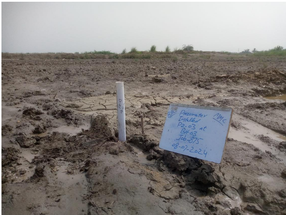
Photo-2: Piezometer installed at the location of BH-03.
