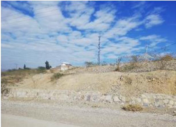
Photograph 6-54: View of telecommunication tower in project area
