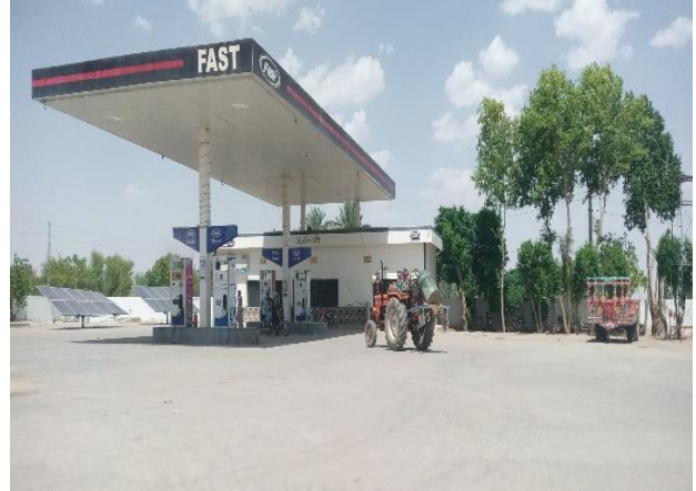
Photograph 6-49: A fuel station within project area
