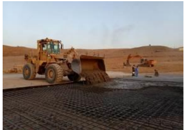
Photograph 4-10: Concrete pouring of rig pad at well site
