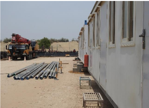
Photograph 4-3: A view of typical rig site mini camp
