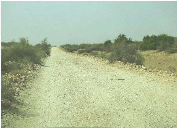
Photograph 4-9: Typical construction of access track
