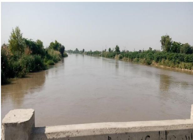
Photograph 6-52: A view of Nara Canal from a bridge within project area
