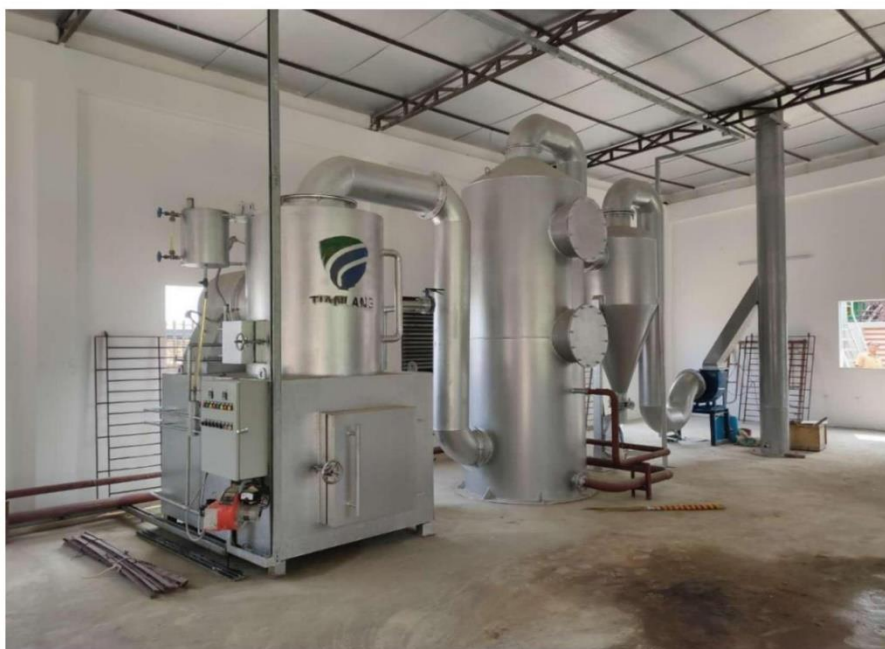
Figure 3-1: Typical Layout of the Plant
