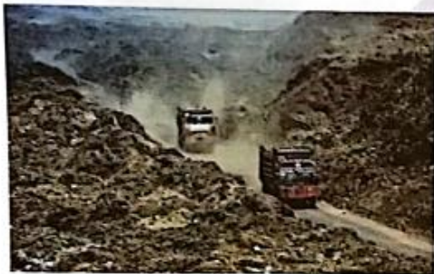
Waste Transportation To LANDFILL SITE
