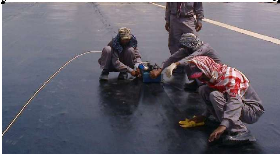
Figure 6.2: Highrise basement water proofing with PVC geomembrane
