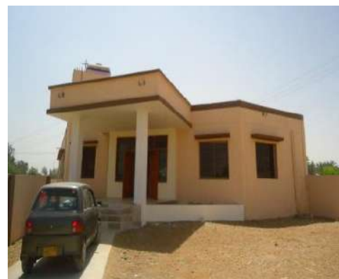
Constructed & Furnished Women Vocational & Skill Development Centre at Kotri, District Jamshoro
