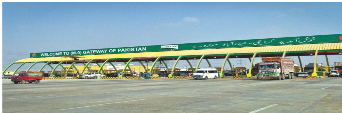
Picture-11: M-9 Motorway
