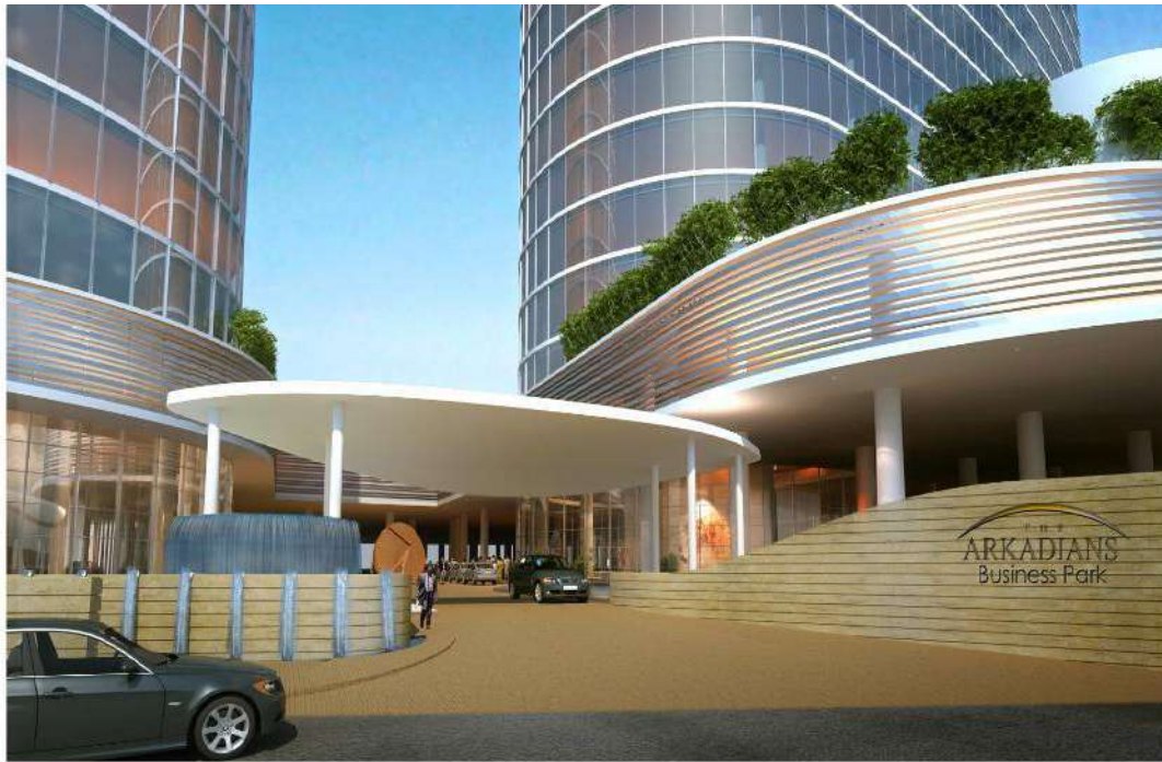
Fig. 2.19: Front View of the Office Towers
