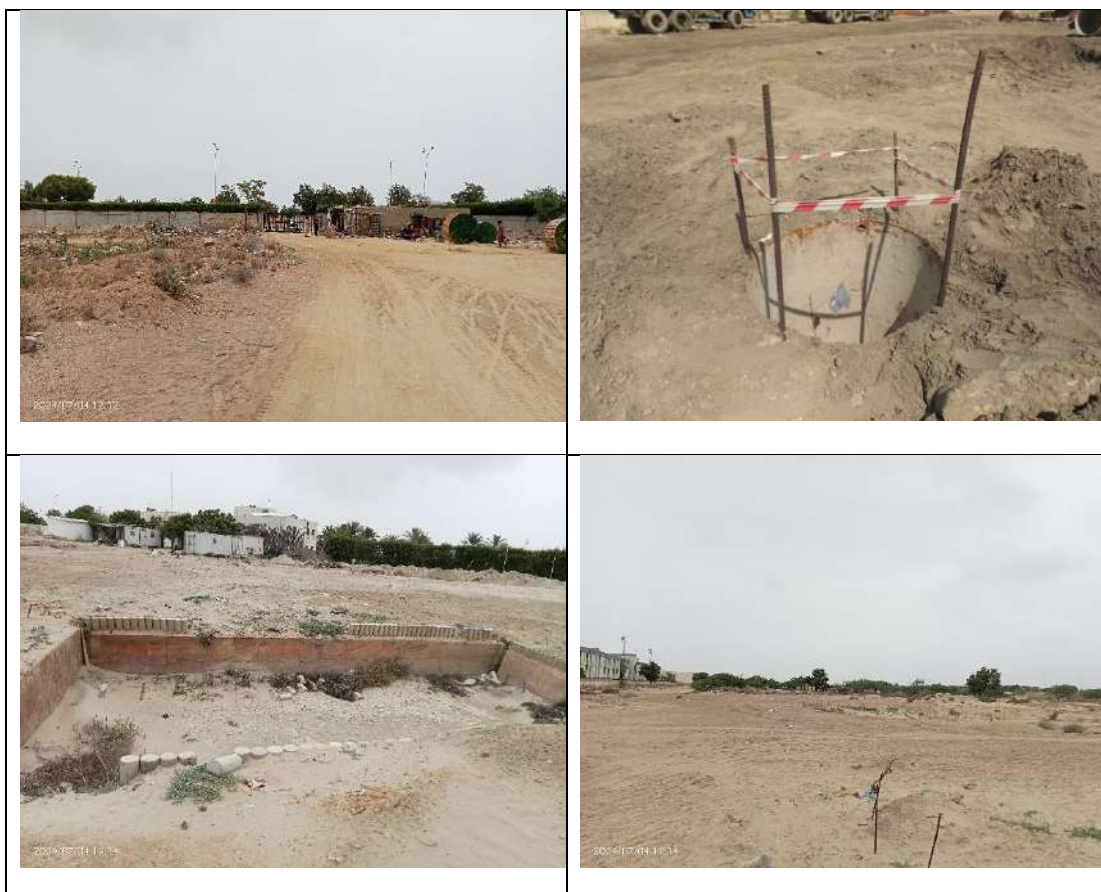
Figure 1-1: Construction site status during Environmental Audit
