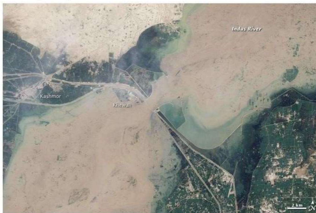
Figure 17: Guddu Barrage Before and After Flood in 2010
