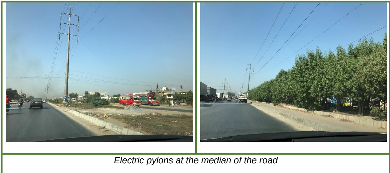
Plate 7.1: Electric Pylons at Median of the Road
