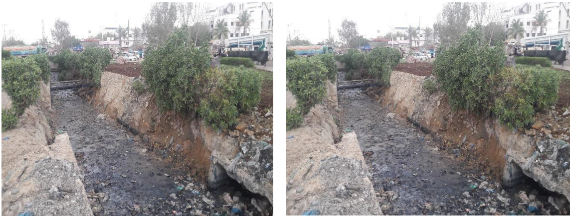
Plate 5.1 Wastewater Drains Crossing Chowrangi at Korangi Road.
